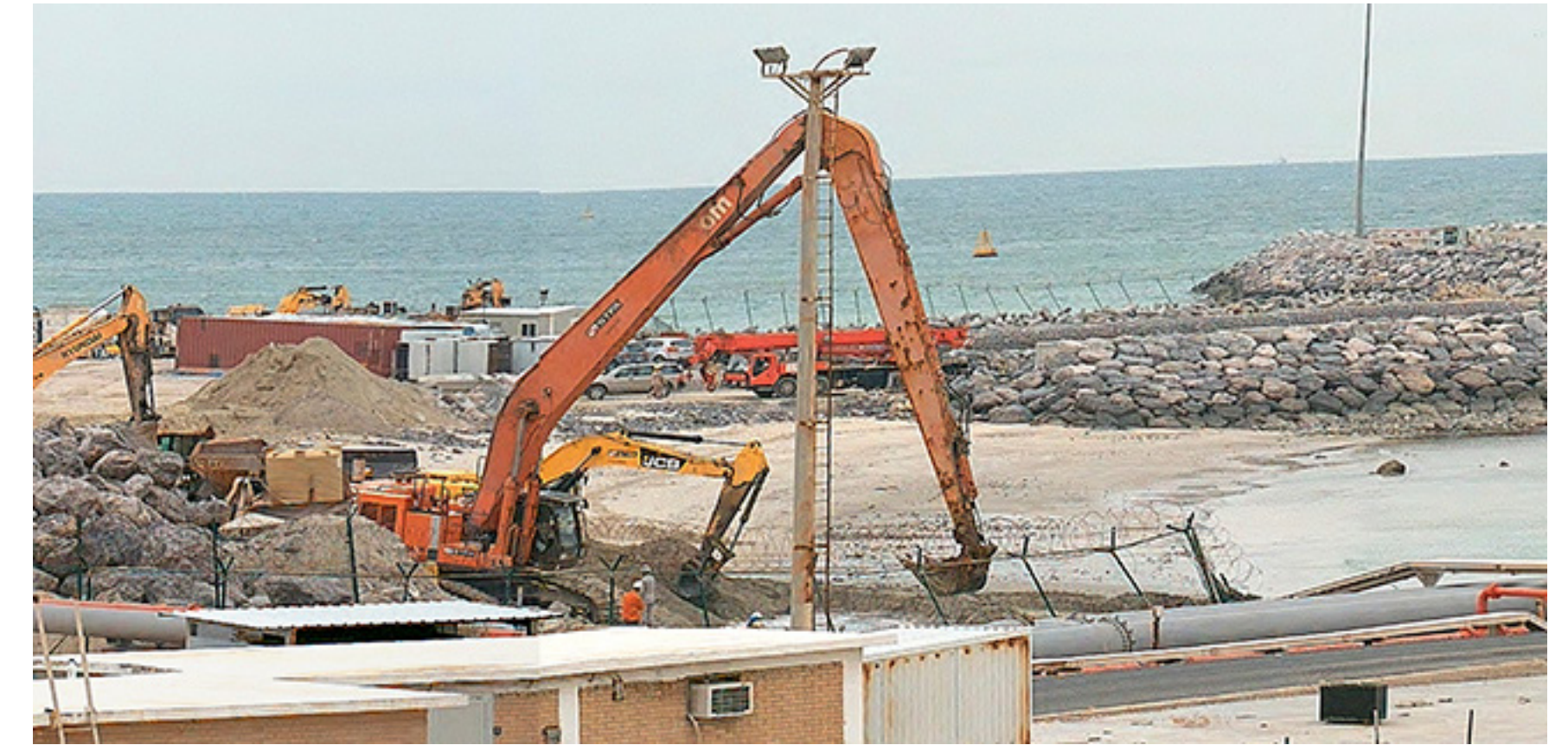
Distance of the excavator: 180 m
